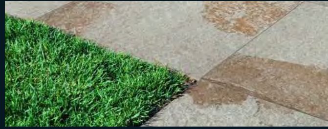
Dry laying on gravel
